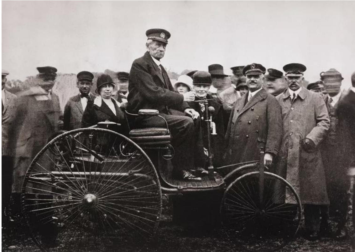
Inventor Karl Benz seated on the 1885 Benz Motorwagen, a three-wheeler called Benz Patent Motorcar. The first patent (DRP No. 37435) for a gas-fueled car on January 29, 1886
