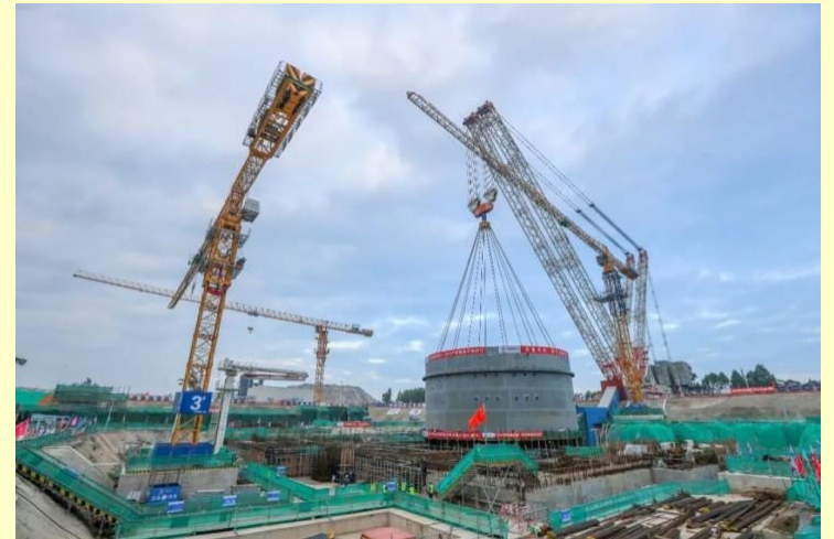
SMR ACP100 construction is in progress
