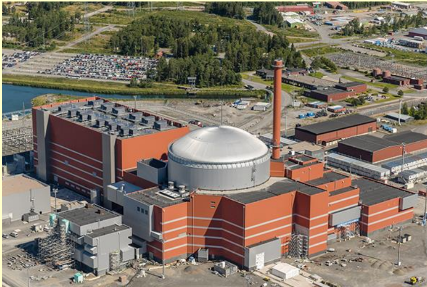
Reactor EPR (Olkiluoto 3)
