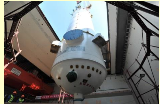
Installation of the HTR-PM reactor (China)
